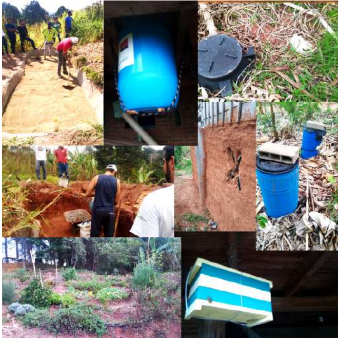
Figure 7: Inconfidentes Campus construction of the ecological septic tank.
