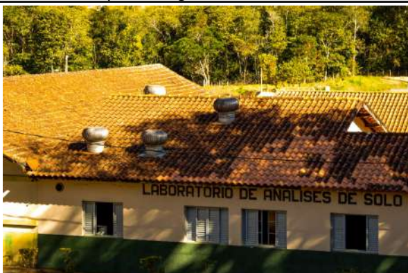
Figure 19: Campus Inconfidentes Soil Analysis Laboratory exhausters.
