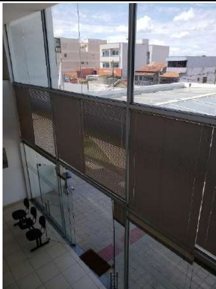
Figure 11: Rectory entrance natural lighting.
