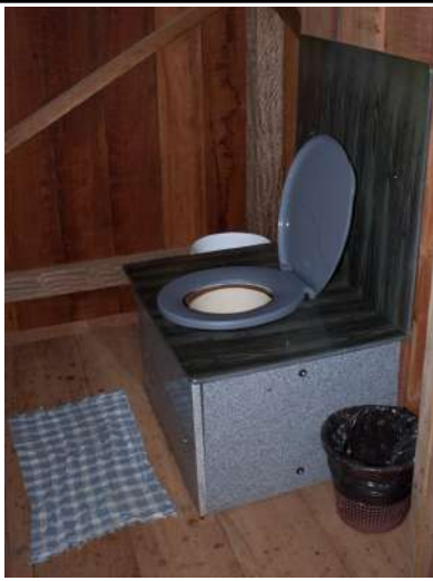
Figure 23: Inconfidentes Campus dry toilet at Agroecology Sector.
