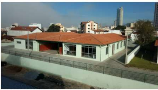
Figure 1: Rectory natural ventilation and lighting
