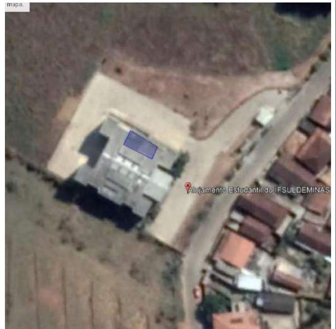
Figure 16. Inconfidentes Campus Solar water heating system.
