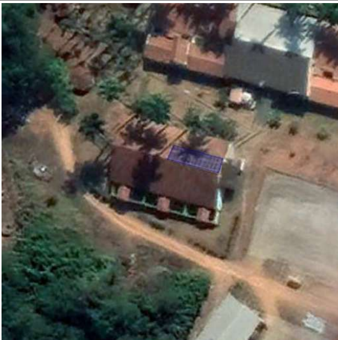
Figure 17. Machado Campus Solar water heating system.
