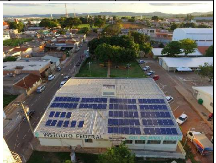
Figure 4: Campus Passos solar power plant.
