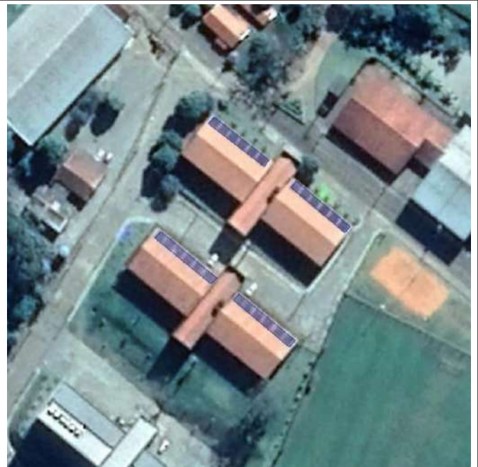
Figure 18. Muzambinho Campus Solar water heating system.
