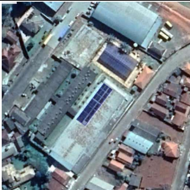
Figure 19. Muzambinho Campus CeCAES Solar water heating system.
