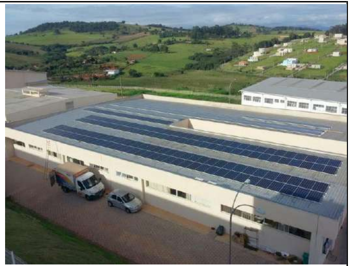
Figure 6: Campus Pouso Alegre solar power plant.
