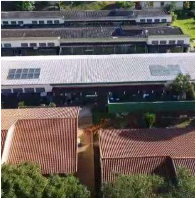
Figure 15. Inconfidentes Campus Solar water heating system.
