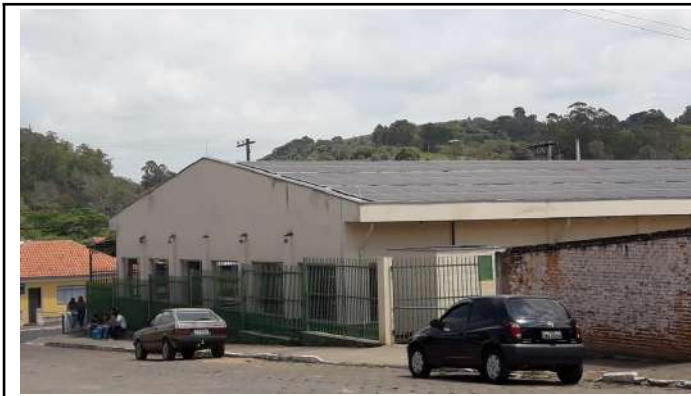
Figure 1: Campus Inconfidentes solar power plant.
