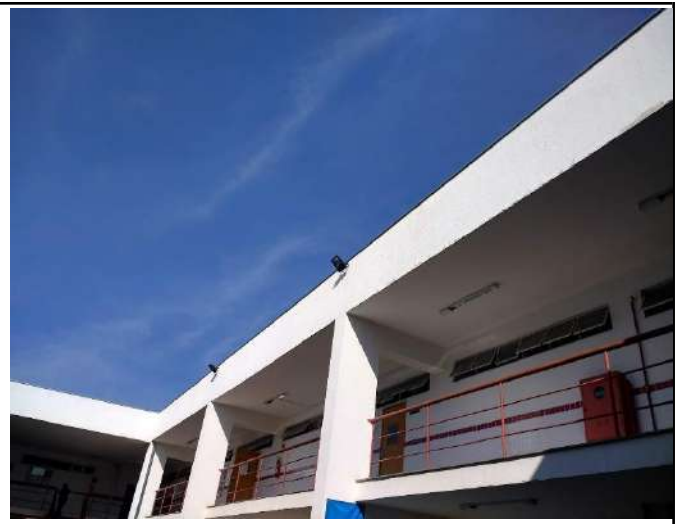
Figure 12: Campus Poços de Caldas high-efficiency luminaires with automatic lighting control – LED spotlights.
