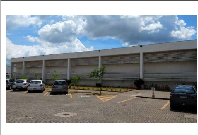
Figure 15: Campus Poços de Caldas shielding adjustment and solar control – Brise-soleil at classroom building.
