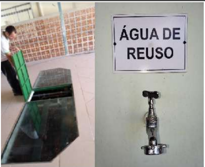
Figure 9: Rectory rainwater recovery system for covering the flushing and irrigation – Water storage tank and reuse water tap.
