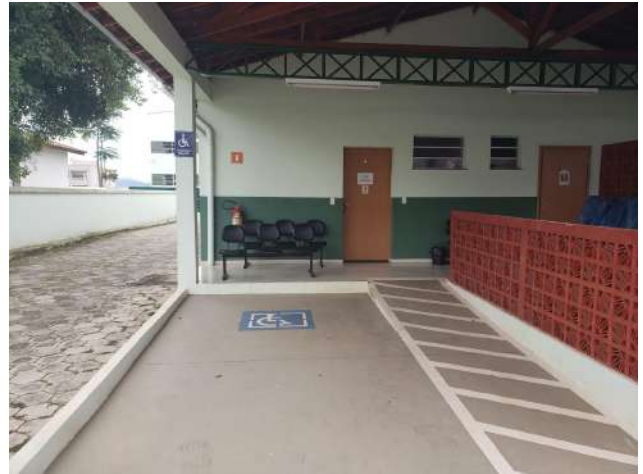
Figure 6: Rectory parking and ramp for people with special needs.
