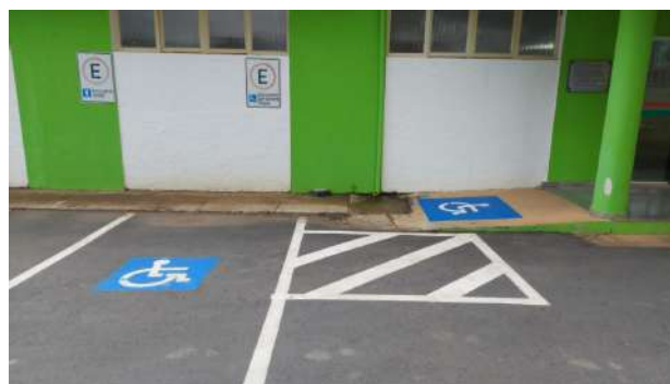
Figure 2: Machado Campus parking ramp for people with special needs.
