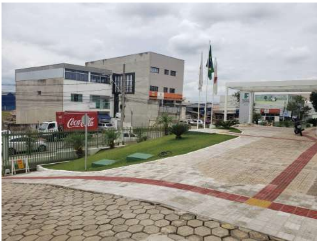
Figure 7: Rectory new tactile paving.
