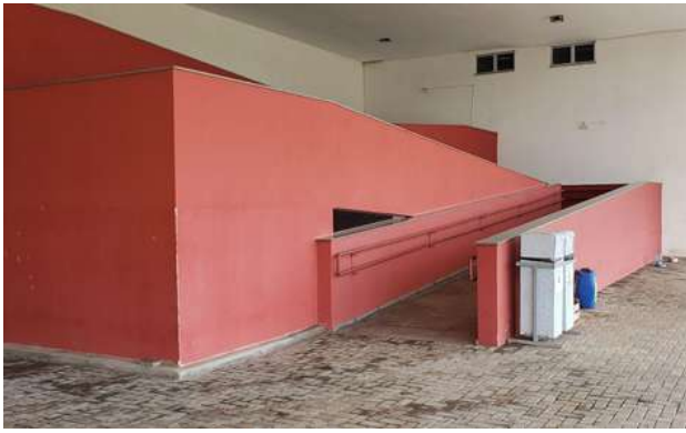
Figure 13: Poços de Caldas Campus ramp and handrails.
