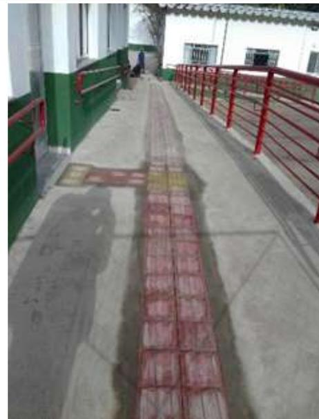
Figure 4: Carmo de Minas Campus tactile paving and handrails.
