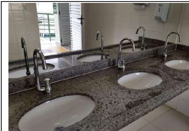
Figure 1: Rectory time delay water taps.
