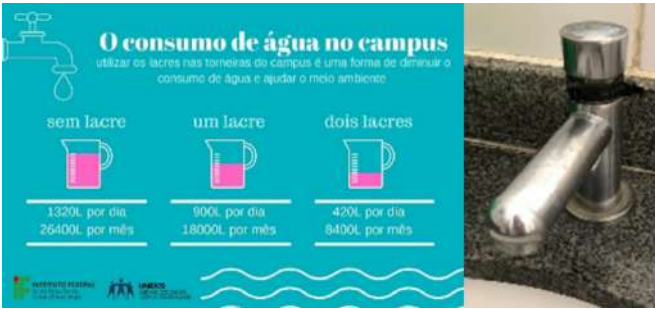
Figure 7: Campus Pouso Alegre tap with cable ties.
