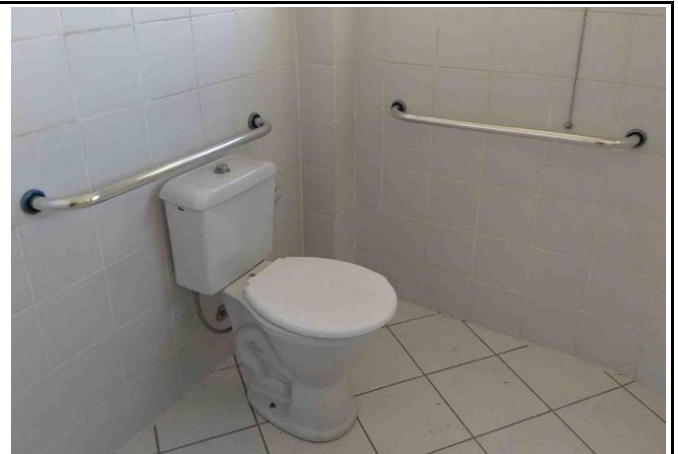
Figure 2: Rectory toilet water box flush.
