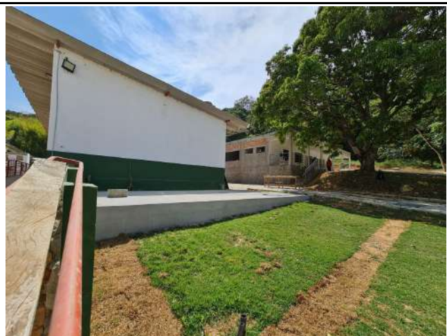
Figure 11: Carmo de Minas Campus space for the installation of rainwater reservoir tanks.
