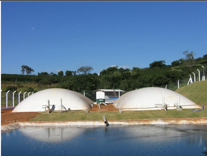
Figure 13. Swine waste treatment unit for biogas production.
