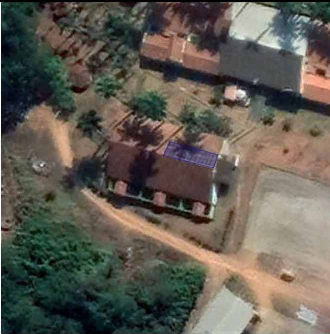
Figure 17. Machado Campus Solar water heating system.
