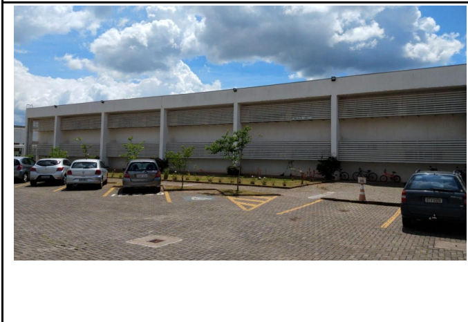
Figure 15: Campus Poços de Caldas shielding adjustment and solar control – Brise-soleil at classroom building.
