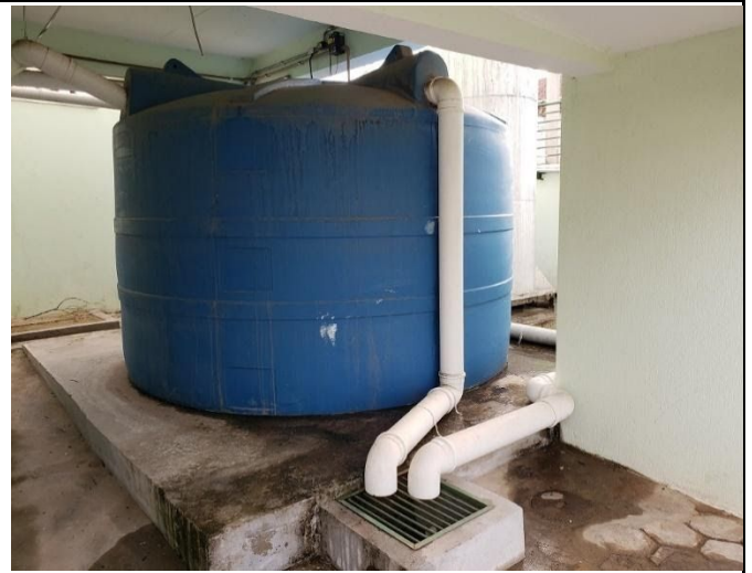
Figure 8: Rectory rainwater recovery system for covering the flushing and irrigation – Water storage tank.
