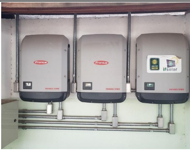
Figure 5: Rectory automatic management system for energy supplies and production – Solar power converters.
