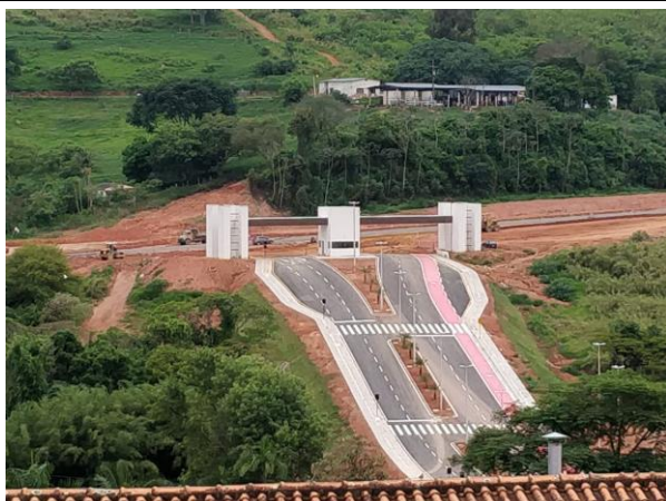
Figura 5 Campus Machado - Road junction construction. Photo taken in 10/31/2018.
