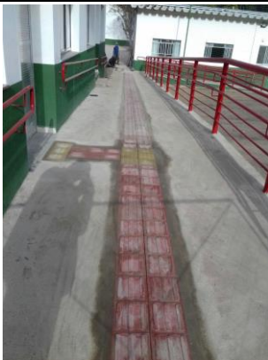
Figura 5 Campus Carmo de Minas - Tactile paving and handrails
