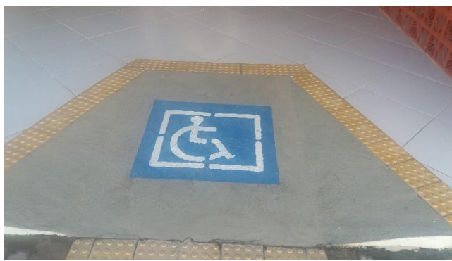
Figura 1 Rectory - Curb ramp
