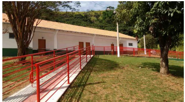
Figura 4 Campus Carmo de Minas - Tactile paving and handrails
