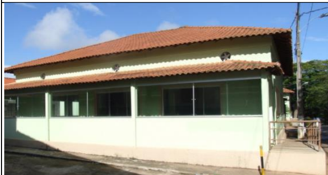
Figura 3 Ventilation – Eolic – Restaurant – Campus Machado
