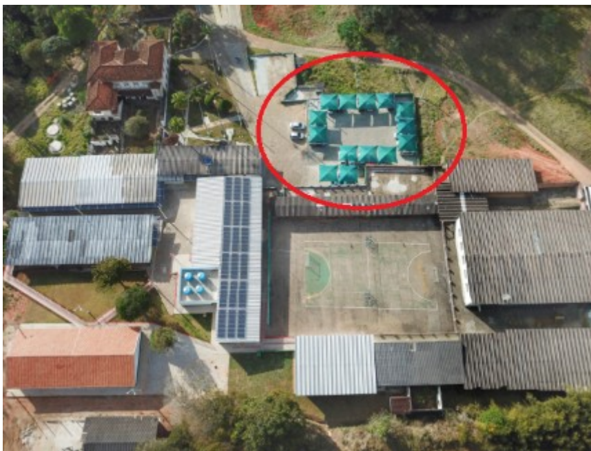
Campus Advanced Carmo de Minas – Parking Lot
