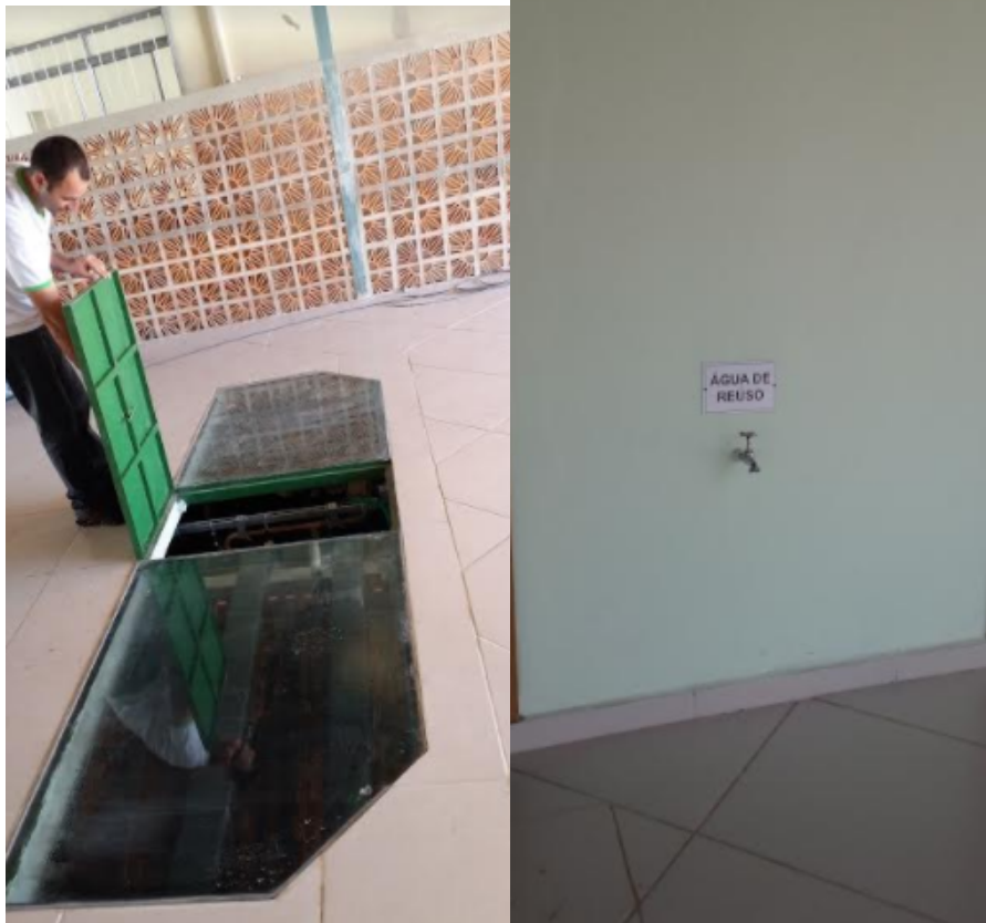
Water Management - Rainwater harvesting system and external water tap for reuse Rectory – Pouso Alegre
