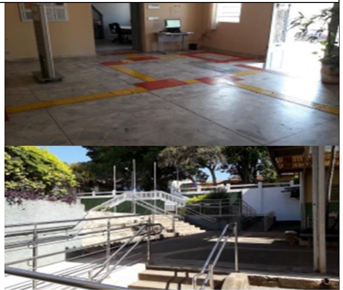
Figure 8: Campus Inconfidentes tactile paving, ramp and handrails.
