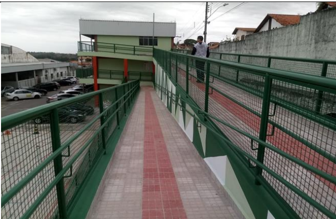
Figure 7: Campus Muzambinho tactile paving, ramp and handrails.
