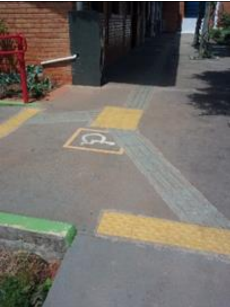
Figure 12: Campus Passos tactile paving.
