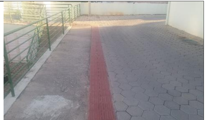
Figure 2: Rectory tactile paving.
