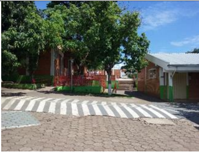
Figure 11: Campus Passos elevated crosswalk.
