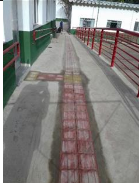
Figure 4: Campus Carmo de Minas tactile paving and handrails.
