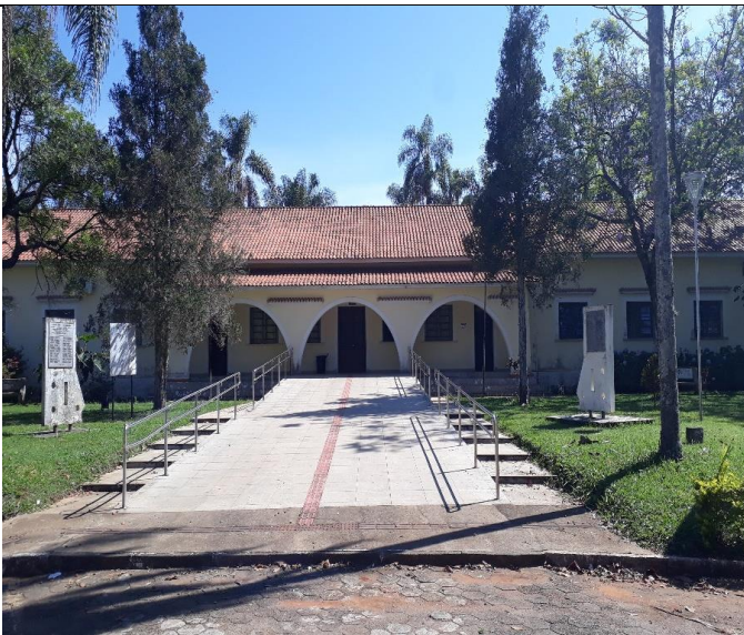
Figure 7: Campus Muzambinho tactile paving, ramp and handrails.
