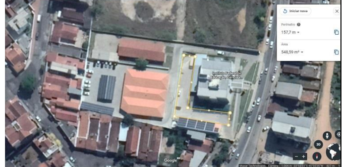
Figure 2: Rectory parking lots.
