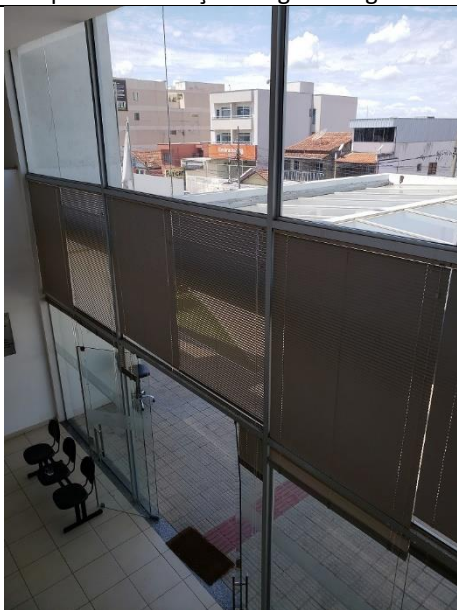
Figure 11: Rectory entrance natural lighting.
