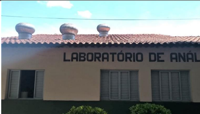
Figure 19: Campus Inconfidentes Soil Analysis Laboratory exhausters.
