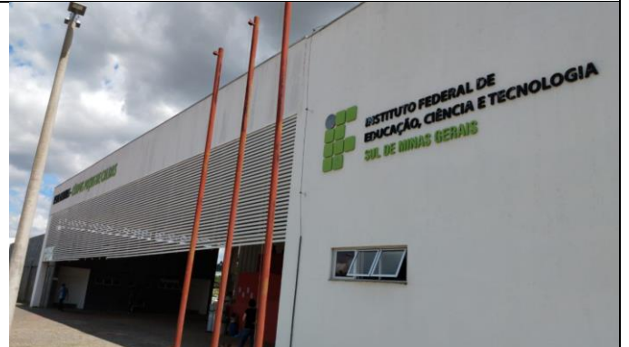
Figure 20: Campus Poços de Caldas building facade brise-soleil.
