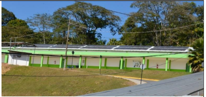
Figure 2: Campus Machado solar power plant.
