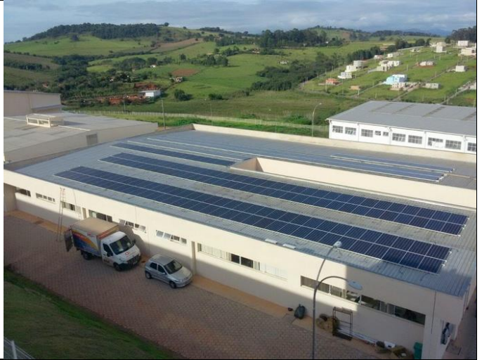
Figure 6: Campus Pouso Alegre solar power plant.
