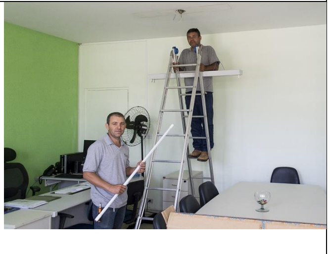
Figure 10: Campus Inconfidentes replacing the lighting in the main building.
